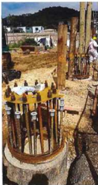
Ground prep for link bridge
