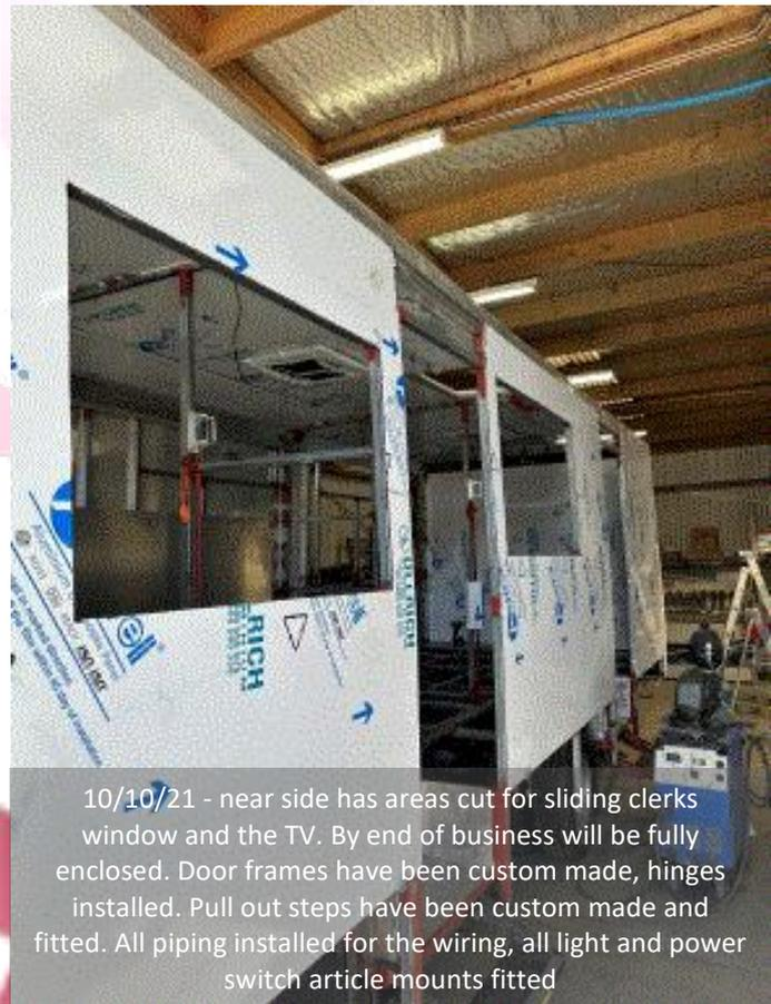
10/10/21 - near side has areas cut for sliding clerks window and the TV. By end of business will be fully enclosed. Door frames have been custom made, hinges installed. Pull out steps have been custom made and fitted. All piping installed for the wiring, all light and power switch article mounts fitted
